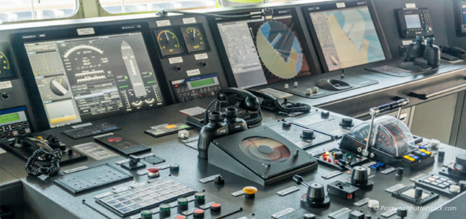
Figure 11: Current state-of-the-art navigational bridge equipment
